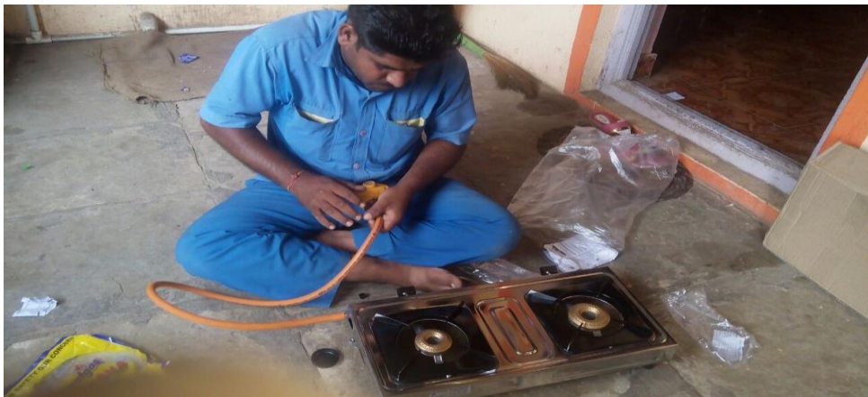
Figure 6.15. Delivery man carrying out leak inspection
